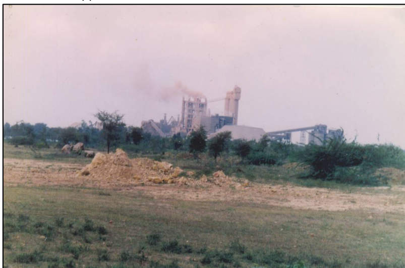
Plate-1.Arasu cement factory –Ariyalur.
